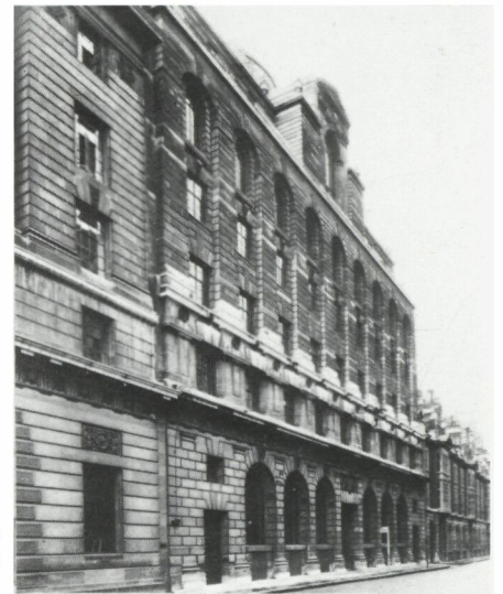
Midland Bank, Princes Street section, completed in 1939.
