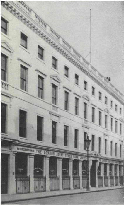
The Princes Street headquarters of the London Bank shortly before the First World War.
