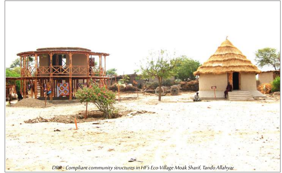
DRR - Compliant community structures in HF's Eco-Village Moak Sharif, Tando Allahyar
